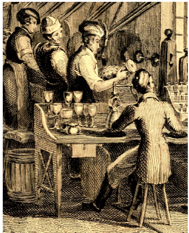
Fig.6 : Detail of glass decorating workshop at Holyrood glassworks, Edinburgh, depicted in 1834, but probably built by 1820. In this workshop the proportion of engravers to cutters was just one to ten. The engraver is using his foot to power the treadle mechanism. Reproduced with the kind permission of The City of Edinburgh Museums and Galleries, The Museum of Edinburgh, and a private lender to the Museum of Edinburgh.
